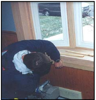
Lightly Sand all Interior Wood Surfaces
