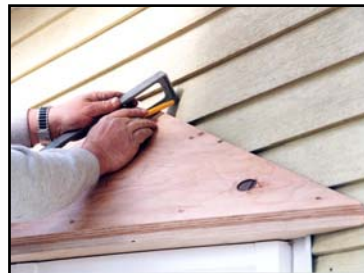
Position Roof Centered on Frame
