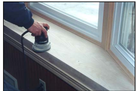
Lightly Sand all Interior Wood Surfaces
