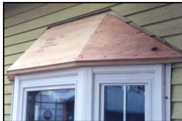
Fasten Roof to Wall and Frame
