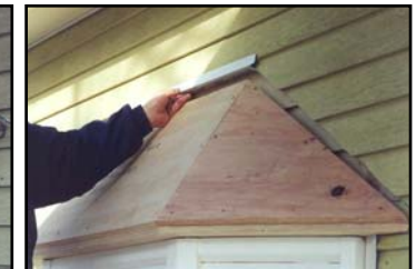
Anchor Upper Eyebolts through Roof
