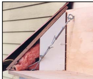
Complete Turn Buckle Hanging System
