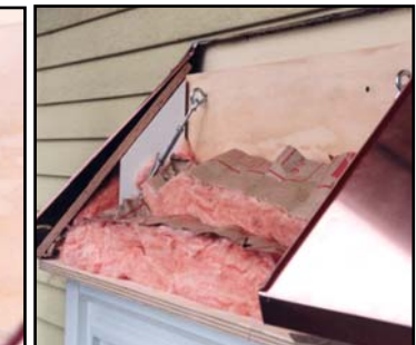
Insulate all Roof Cavities
